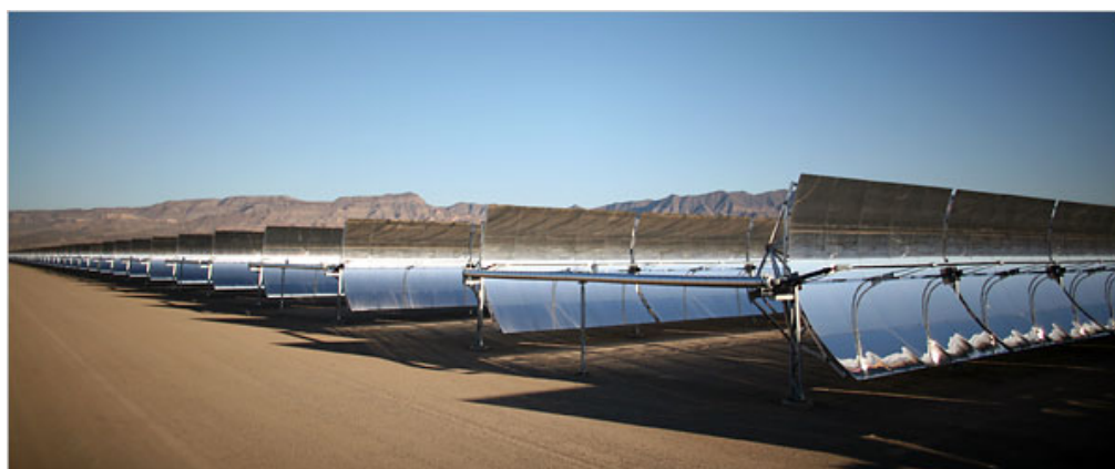
Near Boulder City, Nev., Acciona Energy operates Nevada Solar One, a solar thermal installation with mirrors that gather heat from the sun and convert it into electricity. The plant produces 64 megawatts.
