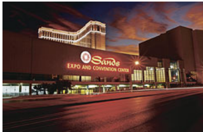
The Sands Expo and the Venetian hotel, background, are part of the new Megacenter.
