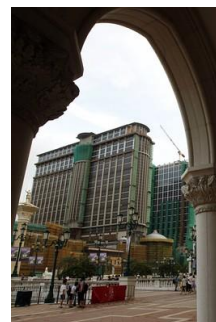
A Sands resort being built on Cotai
