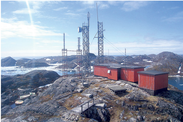
ADS-B receiving antennas have been installed in Greenland to receive flight information from trans-Atlantic airline flights.
